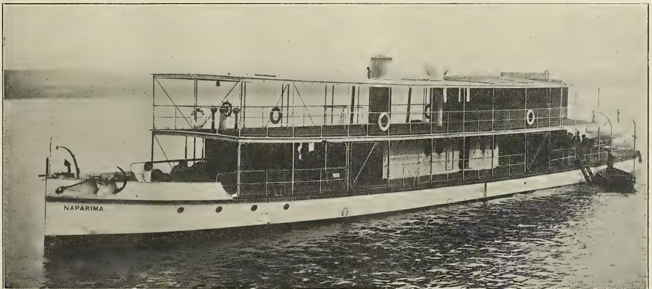
THE NAPARIMA, A TYPICAL SHALLOW-DRAFT, SCREW-PROPELLED STEAMER
